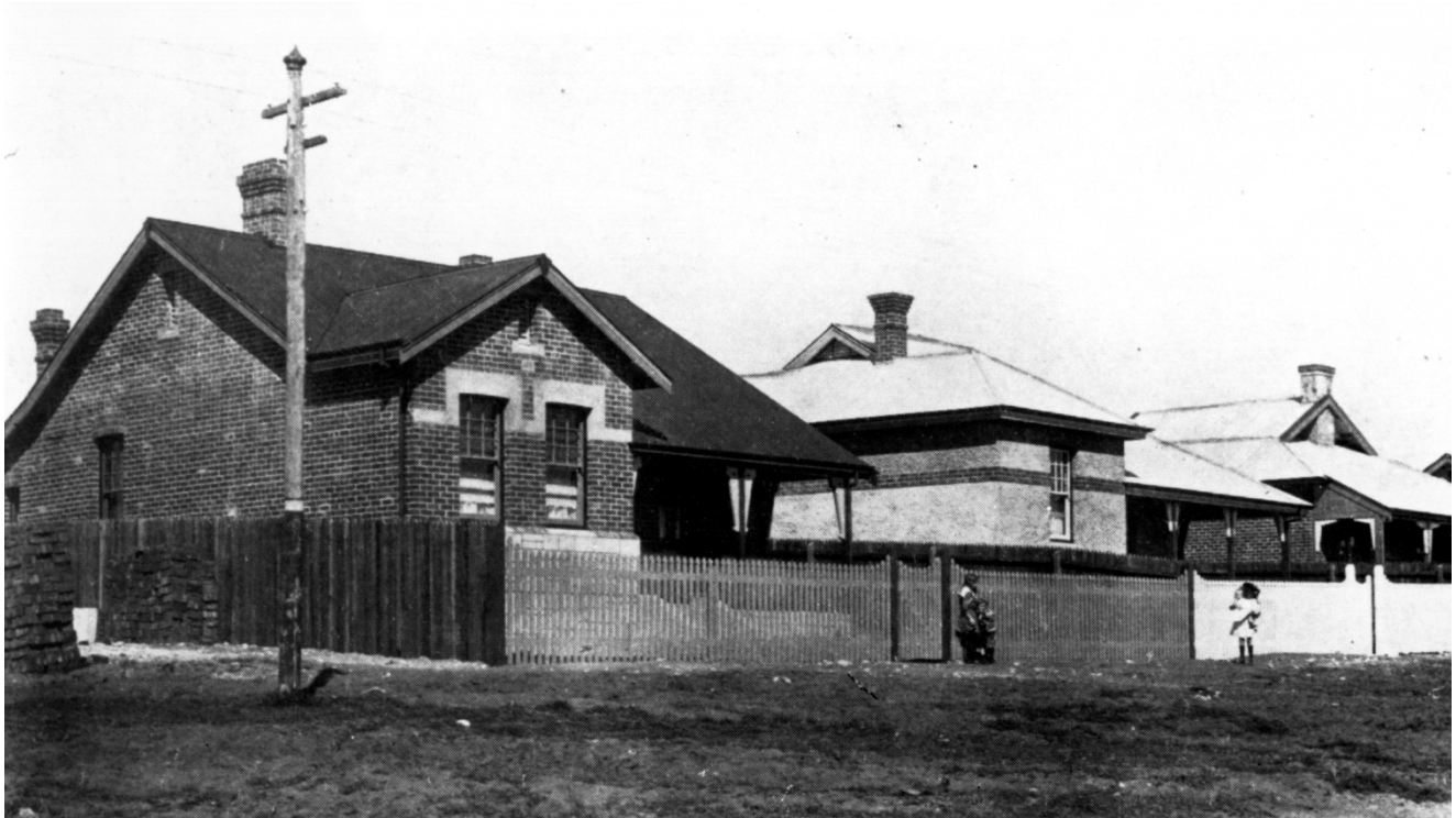
First Fremantle Housing Board houses under construction, No 41 Forrest St is at left. Workers Homes Board, 1913 (detail).
